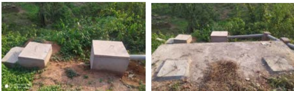
Figure 4: Three stage treatment of laboratory waste
